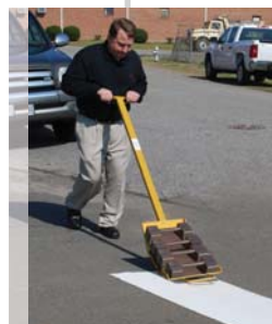
Installation with a tamper cart using 270 ES for a stop bar.
