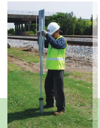
Anchor installation with a Universal Slide Hammer
